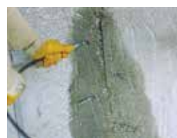
Hose set coupling to installed mechanical packer.
