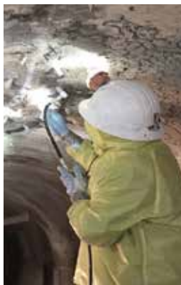
Over Head Injection with Button Head Packers
