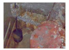
Figure 1. Vault Water Infiltration
