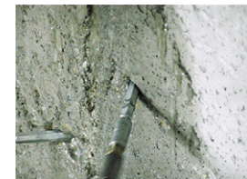
Port placement at 45 degree angle.
