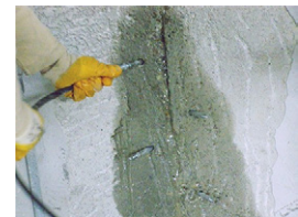
Hose set coupling to installed mechanical packer.
