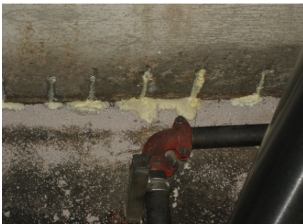
Figure 1. Drill hole placement
